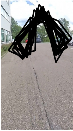
(a) Without stabilization
